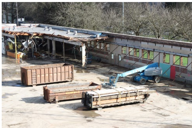
Above: Bound trailer loads of timber salvaged from demolition for Benson Tech modernization. They will be recycled for other uses.
